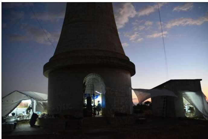
Pre-dawn: MEG, lighthouse and gas house.
