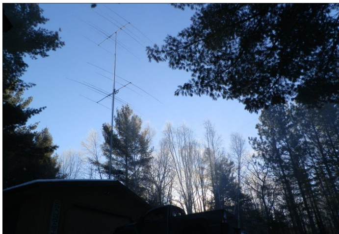
Two Force 12 C4/C3 at 82 ft and 55 ft on a US Tower 71-ft tubular power-up tower, with an 11-ft mast.
