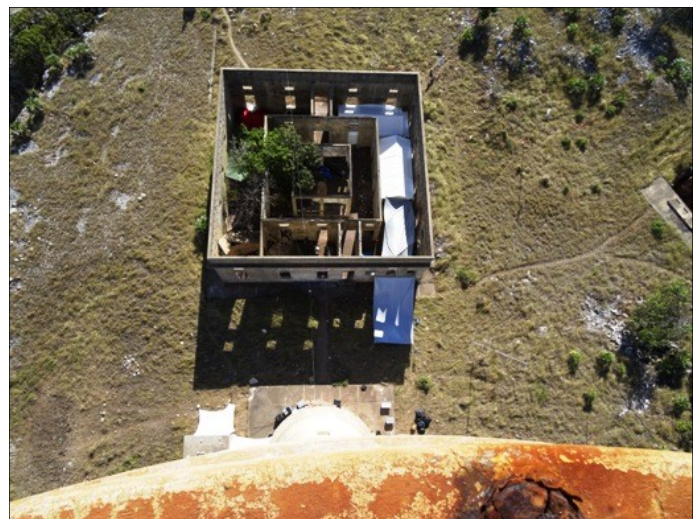
Looking down on the keeper's house.
