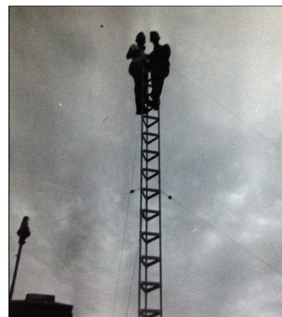
Ron, K8OAN and I installing Rohn 6 tower at my parents house.
