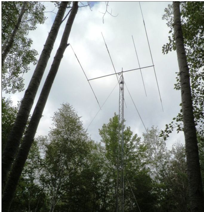
The rebuilt A4 on a 56-ft Rohn 25 tower, which is located 350 ft away, back in the woods.
