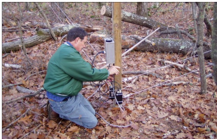
The two bi-directional Beverage antennas require yearly maintenance.
