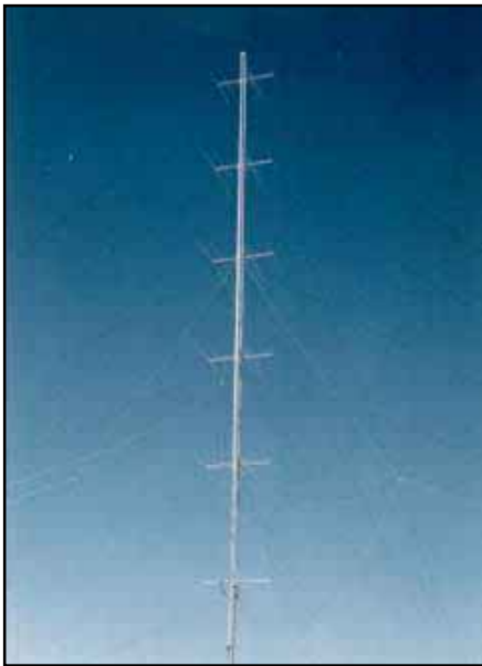
A stack of six Force 12 C-3s (30 to 180 feet) on a 190-foot rotating tower at N7ML.
