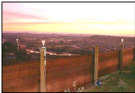
A triangular, phased kW Illuminator "array."
